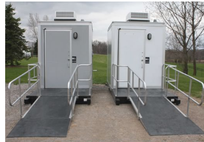
Accessible, mobile outdoor restrooms at a shelter site
